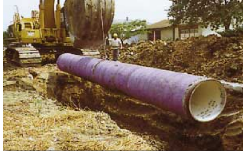
The San Antonio Water System (SAWS) has created a separate recycling water delivery system with approximately 73 miles of transmission trunk lines.
